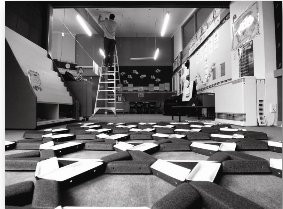
Figure 12: Preparing the ceiling of School A for suspension of the 'Tri-Form'
